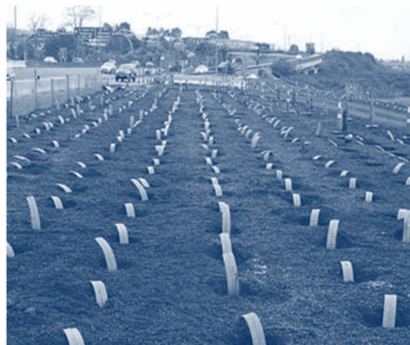
Figure 4.1.4e: The installation of PVDs at our project sites to improve the soil condition and the safety of our operations.
