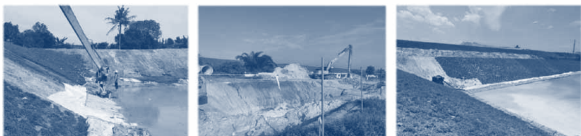
Figure 4.2.1c: We constructed a sediment basin for flood mitigation at Kampung Damai, Sungai Buloh.
